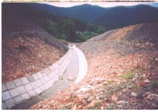
Photo 8. The finished guard channel
