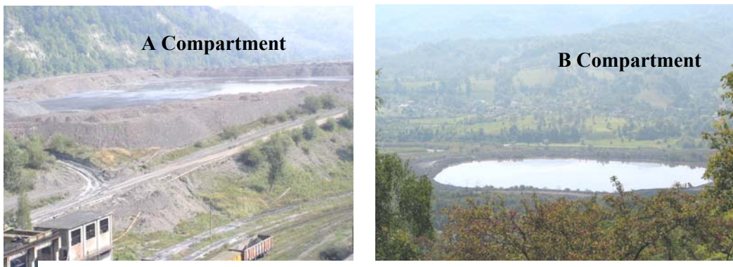
Photo 3. No 1 settle pond with 2 compartments (A and B)
