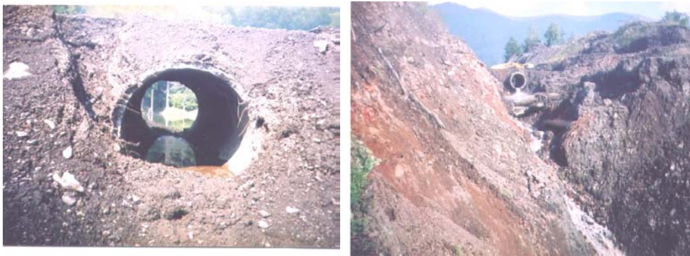
Photo 6. Concrete tubs introduced at gap's limit
